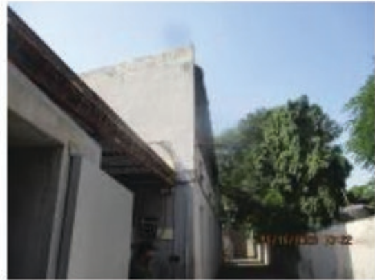
Overview of building.JPG
